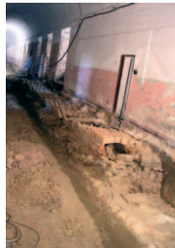
Fig. 8. Kutná Hora, Jesuit College. East wing interior. Stone dewatering shaft. Surface part with numerous younger events visible. Shortly after 1667. View from the north.
