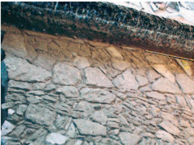
*Fig. 17.* Kutná Hora, Jesuit College. Upper courtyard. Part of the stone facing damaged by the building's transformation into a barracks (after 1776). View from the south.
