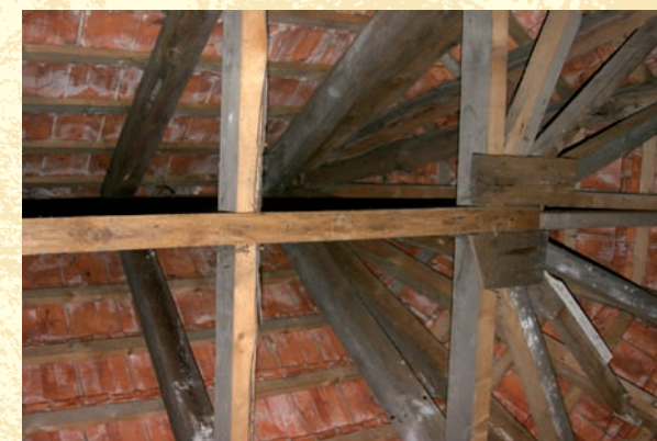
View of the chapel roof truss.
